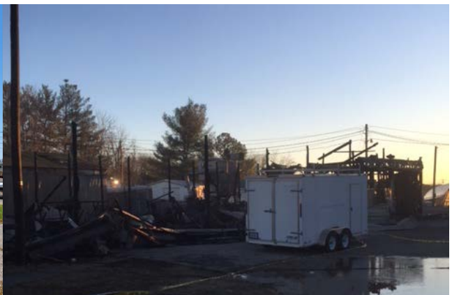
Southwest View After Fire
