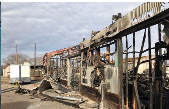
Southwest View After Fire
