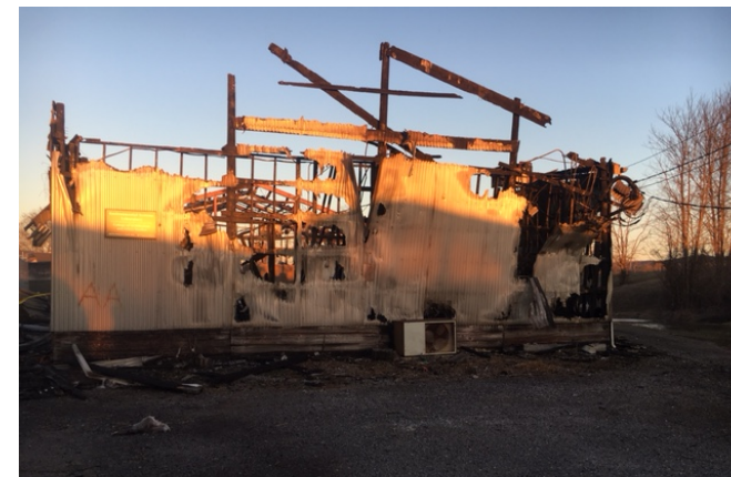
East View After Fire
