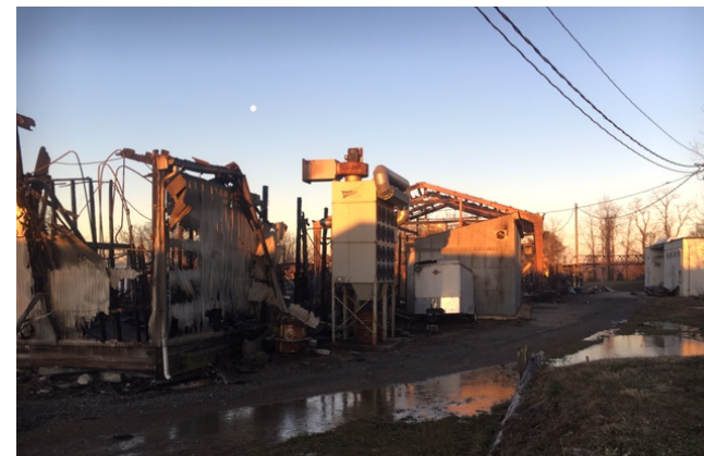
Northeast View After Fire
